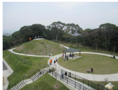
①延命配水池[新展望所]
